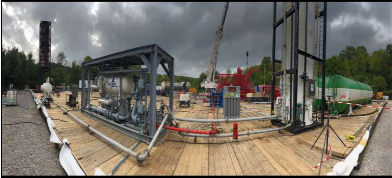
Figure 4: Example Well Testing Package. Shown: Choke Manifold, Well Testing Separator, flare stack, surge tank and Wellhead. [15]
